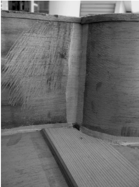
Figure 3. Tool marks on the inside of the ribs.
